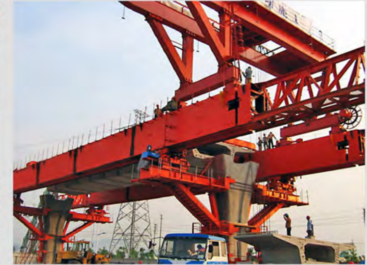
Underslung Segmental Launching Gantry
