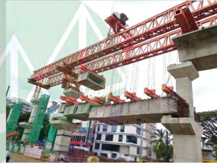
Overhead Segmental Launching Gantry
