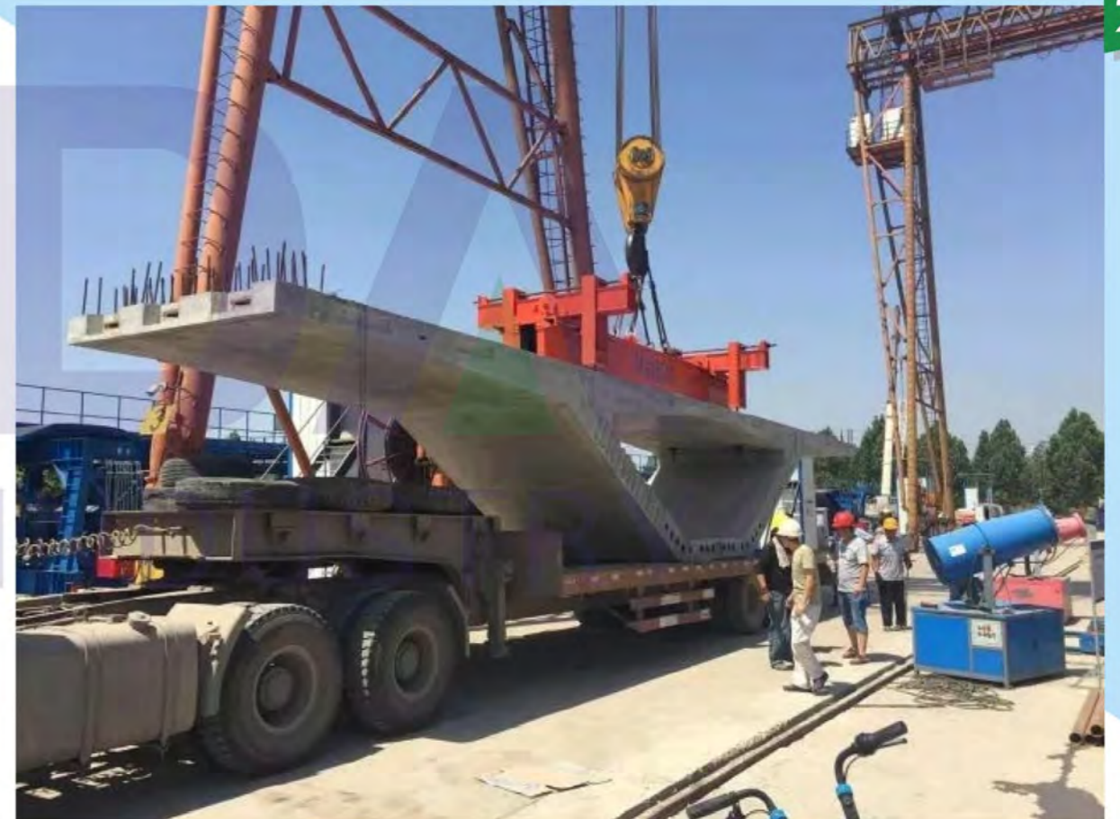
Short Line Method Precast Segment Mould
